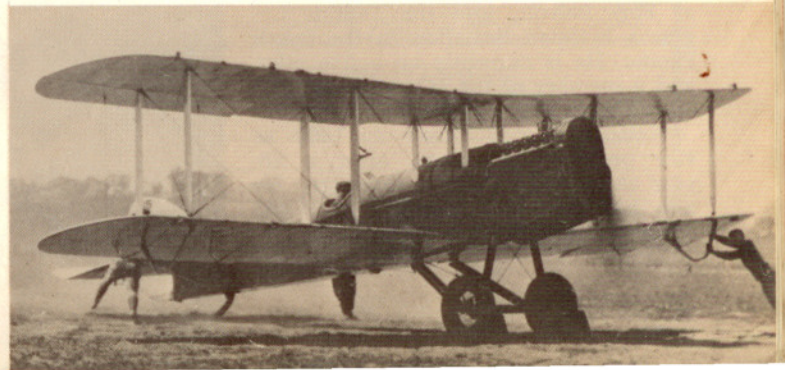
The de Havilland DH-4, a converted World War I type, was the mainstay of the Post Office fleet through 1926. As shown by the men around it, this airplane was big: wing span, 42 feet, 5½ inches; length, 29 feet, 11 inches; and height, 11 feet. Gross weight was 4,595 pounds, and cruising speed was 104 m.p.h. with up to 500 pounds of mail.
